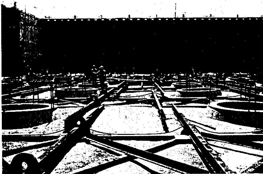
Fig. 12--Detail of the foundation slab placed underwater: top of trestles immersed in concrete
