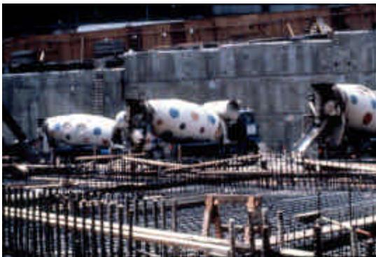
Fig. 8. Placement of self-compacting concrete in a reinforced slab foundation of a skyscraper (Commercial Center) in New York (1978)
