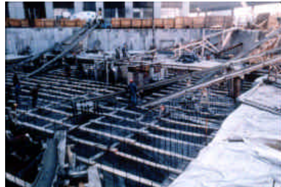
Fig. 9. Placement of self-compacting concrete only chutes for the slab through foundation of the Trump Tower – New York (1978)
