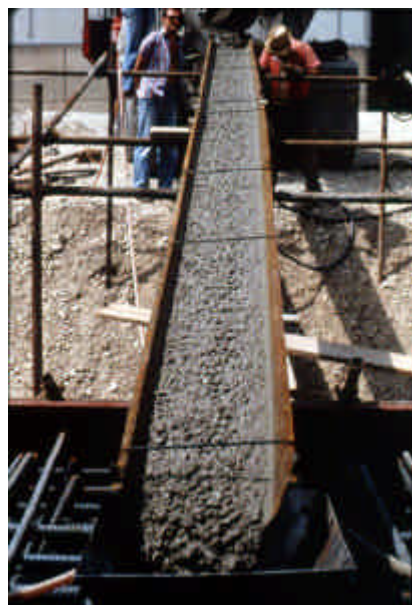
Fig. 6 - Self-compacting concrete placed by chute [8].
