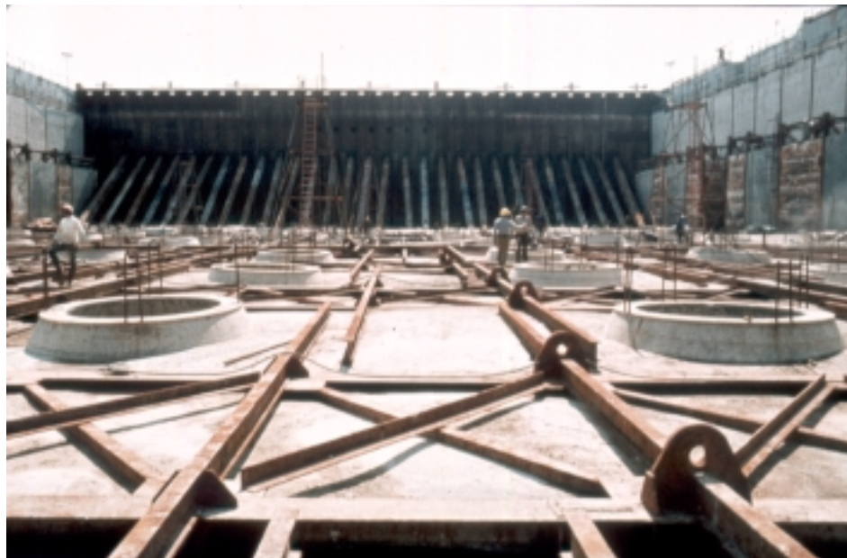
Fig. 4 - View of the reinforced slab foundation placed under water without vibration [4].
