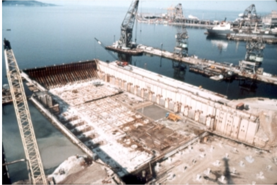
Fig. 3 – Aerial view of the dry dock after removing sea water [4].
