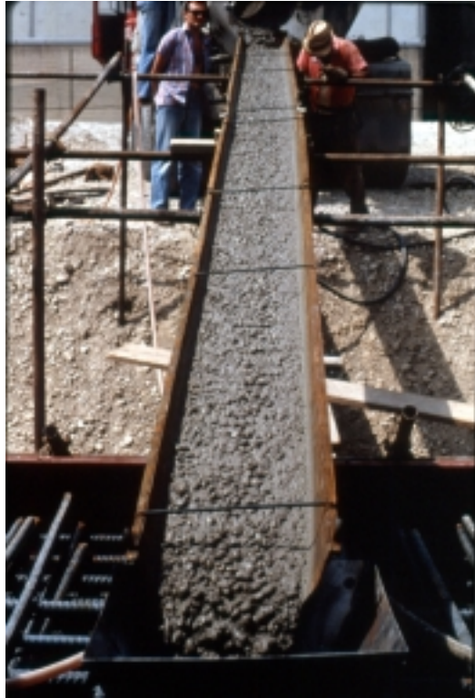
Fig. 5 - Self-compacting concrete placed by chute [8].
