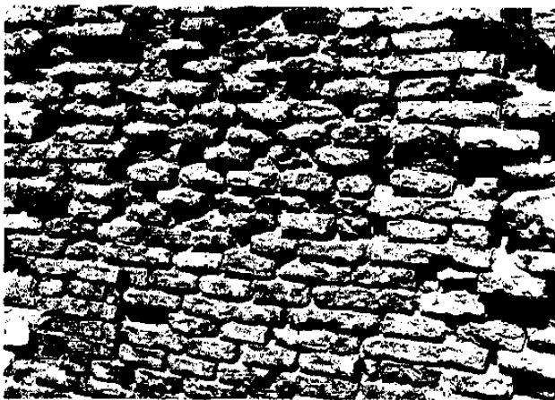
Fig. 2 Deterioration of bricks and jointing mortars.
