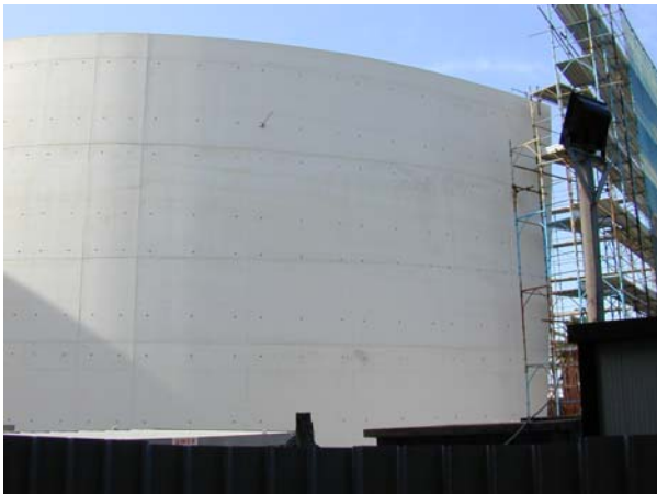
Figure 2 . View of a white wall of the S. Peter Apostle Church in Pescara (Italy).
